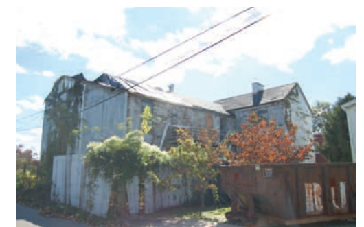
Rear of 151 Constitution pre-renovation
