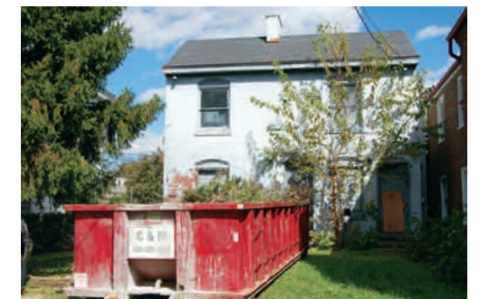
Exterior of 151 Constitution pre-renovation
