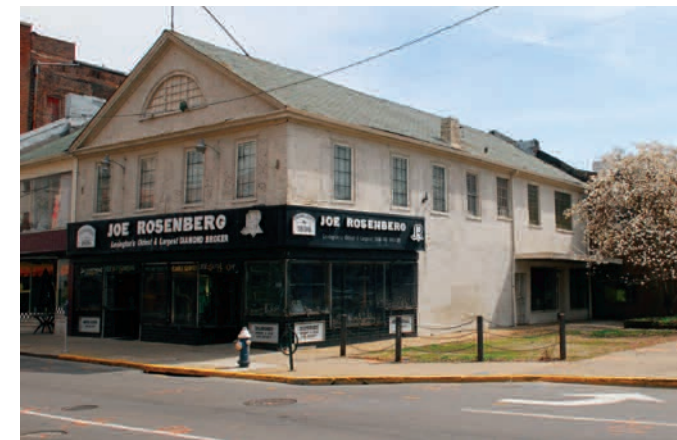
Upper Street pre-demolition
