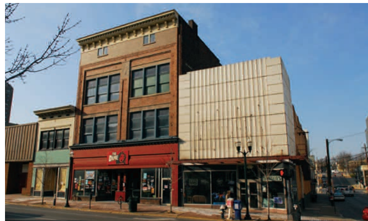
The Dame and Busters pre-demolition
