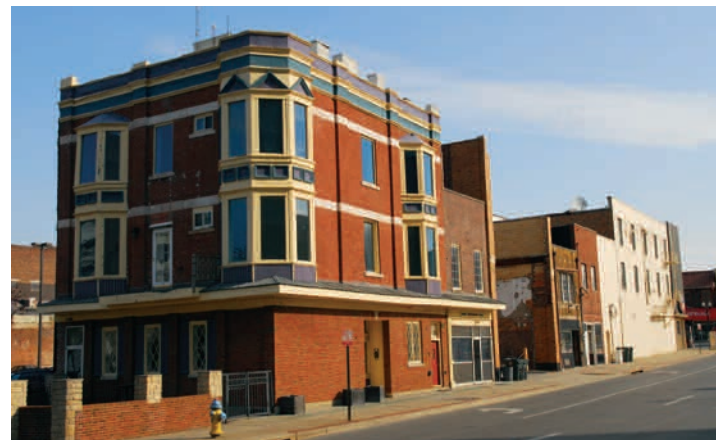
The corner of Vine and Limestone pre-demolition
