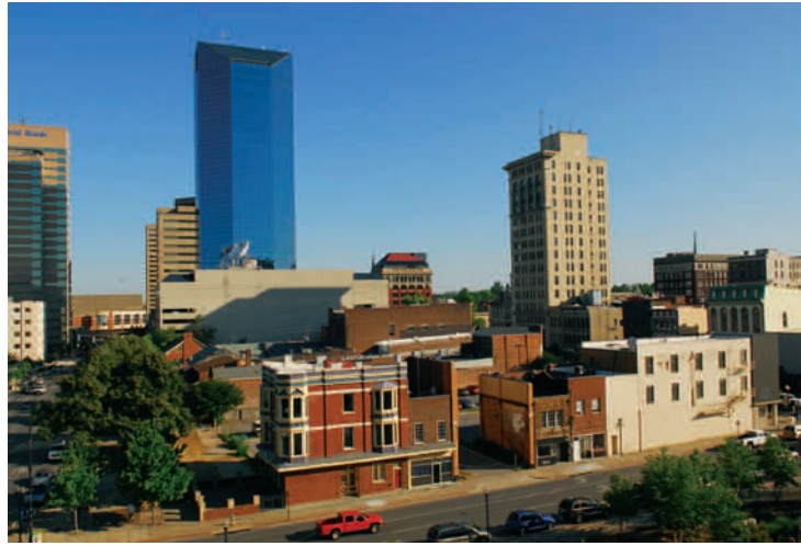
Skyline view of city block along Limestone pre-demolition
