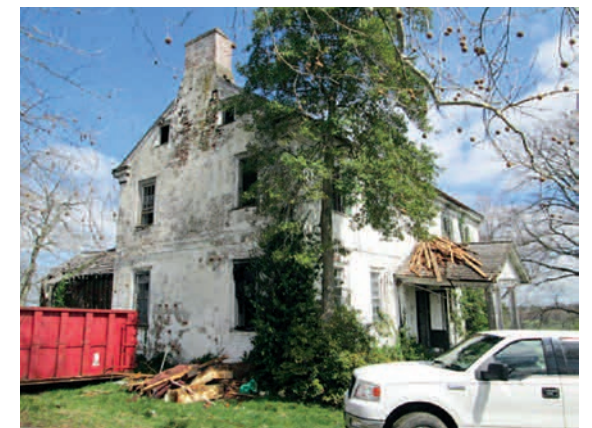
Robert Sanders house as demolition begins
