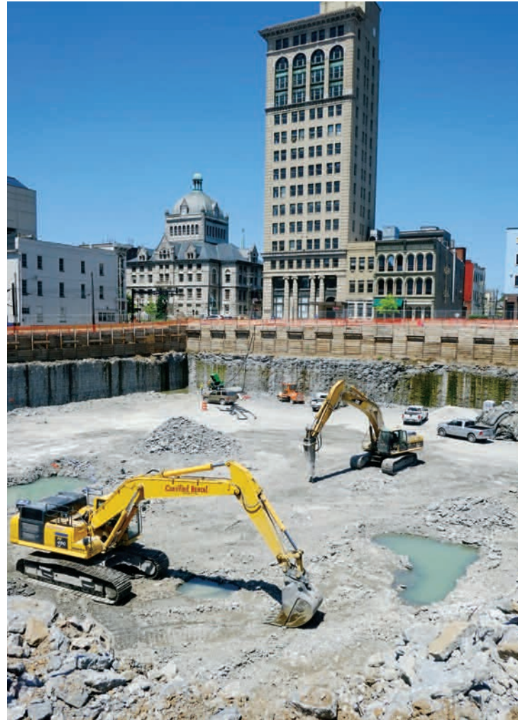
The pit at CentrePoint
