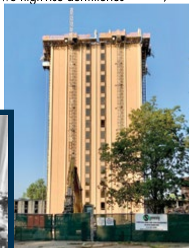
Above: Blanding Tower, the former University of Kentucky residential hall, being demolished a floor at a time Left: Dining in the Commons Cafeteria in 1986 at the Kirwan-Blanding Complex" (University of Kentucky photo)
