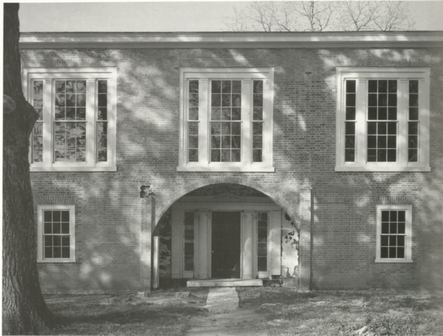
Fig. 6.42. (Above) Pope Villa Facade in 2002; partially restored (portico missing). (Michael Freeman photograph). (Opposite) Pope Villa facade in 2005 with Latrobe version of the portico restored. (© Scott Heisy, 2005)
