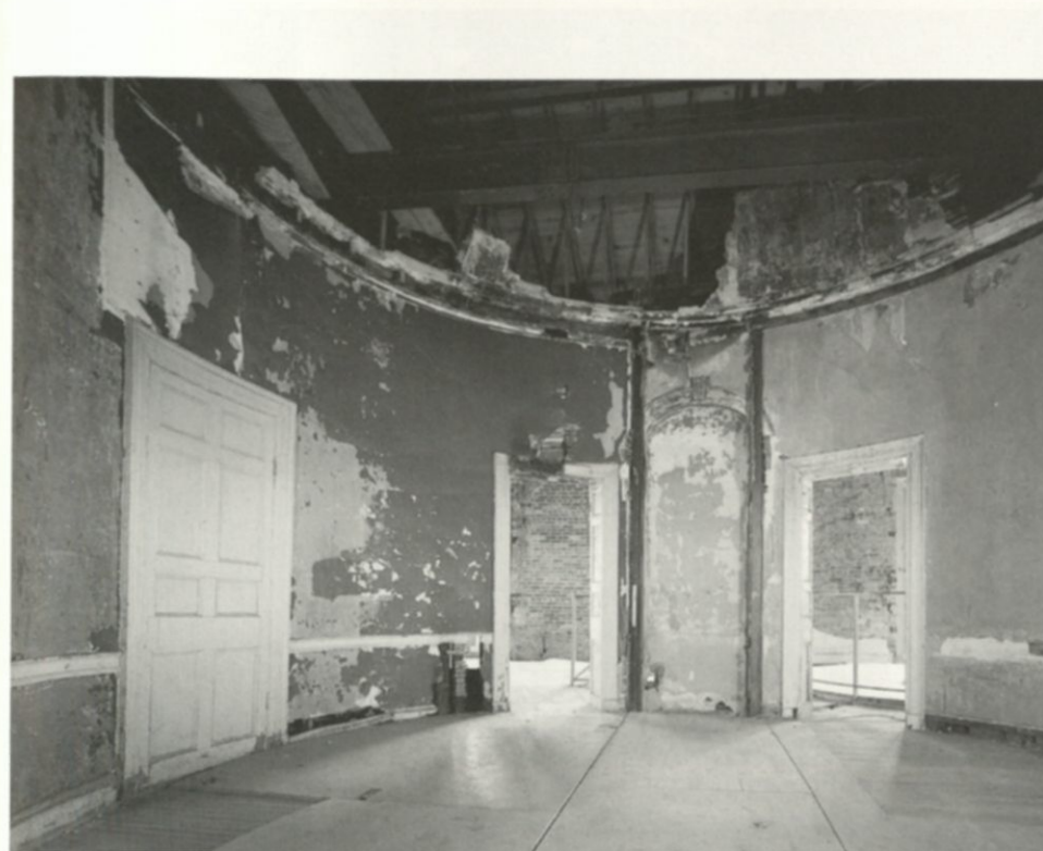
Fig. 6.46. Pope Villa rotunda interior, looking north toward the twin doors of dining and drawing rooms (2002 photograph shows the effects of the 1987 fire and subsequent conservation work; the plaster and wood dome was almost entirely destroyed). (Michael Freeman photograph)
