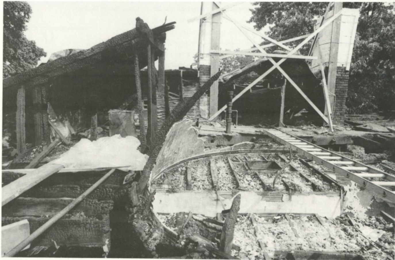
Fig. 6.58. Photograph of Pope Villa attic and roof after fire of 1987. Remains of dome and rotunda (center) with early twentieth-century partitions and ceiling; beyond, temporary wooden bracing of chimneys after fire. (Patrick Snadon, 1987)
