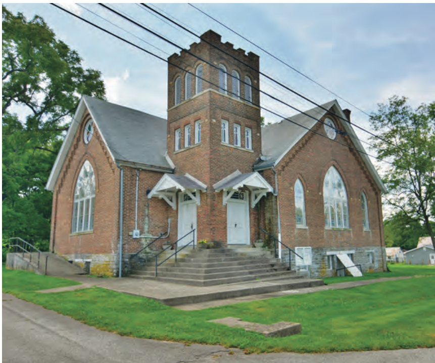
CME Church in Millersburg, Bourbon County. Go to the full Rehabilitation Opportunities list on our website to find out more about the unique history of the materials used to build this church.
