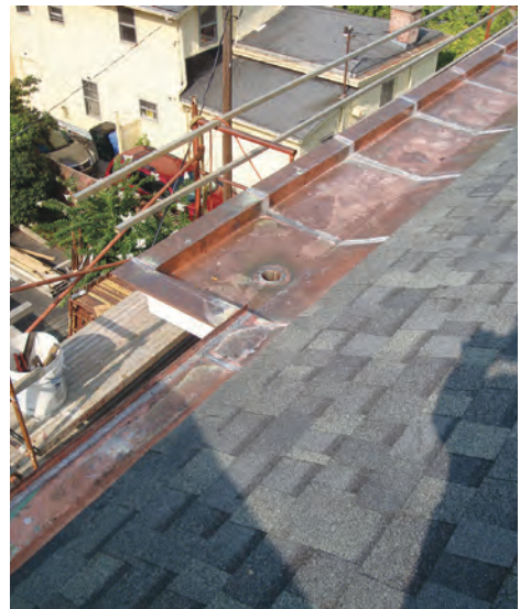
New copper box gutters
