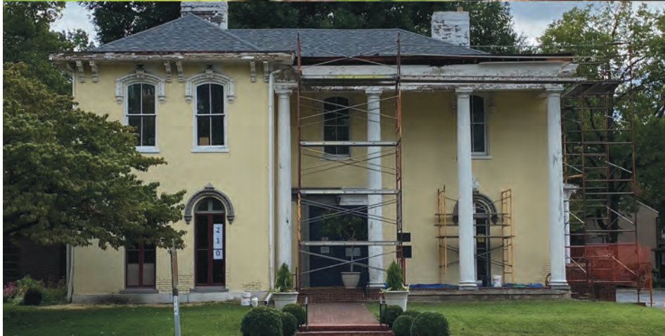
Restoration in progress
