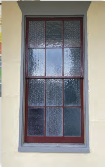
Completed window restoration
