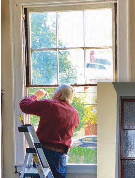
Each window is removed, restored, and reinstalled
