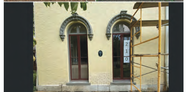
Stages of window restoration
