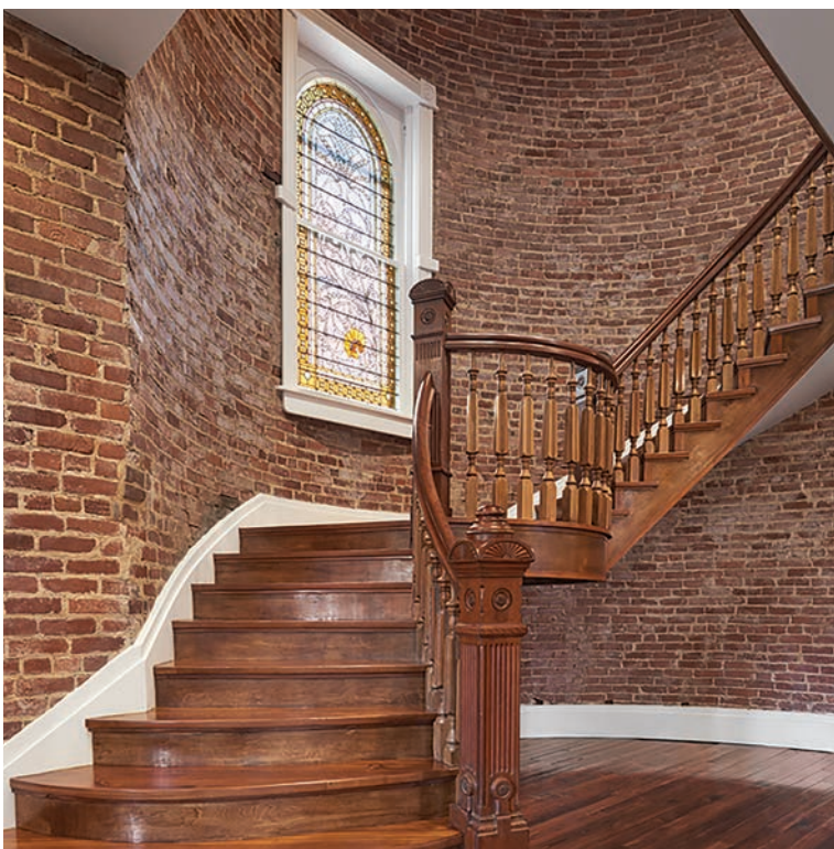
View of the rebuilt stairs and the refinished heart pine floors
