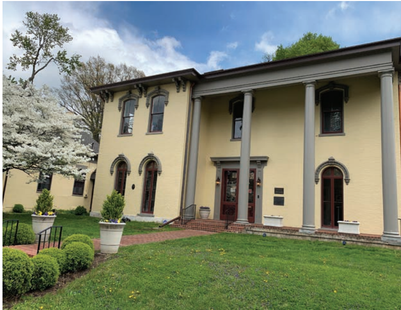
The Dr. Thomas Hunt Morgan House renovations 98% complete
