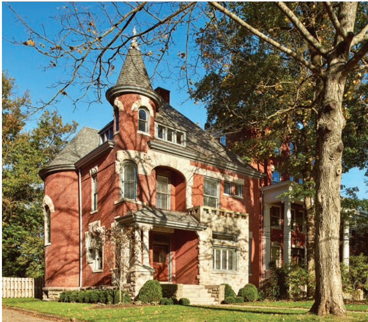
445 West Second after renovations were completed (Courtesy of GLINT Studios)
