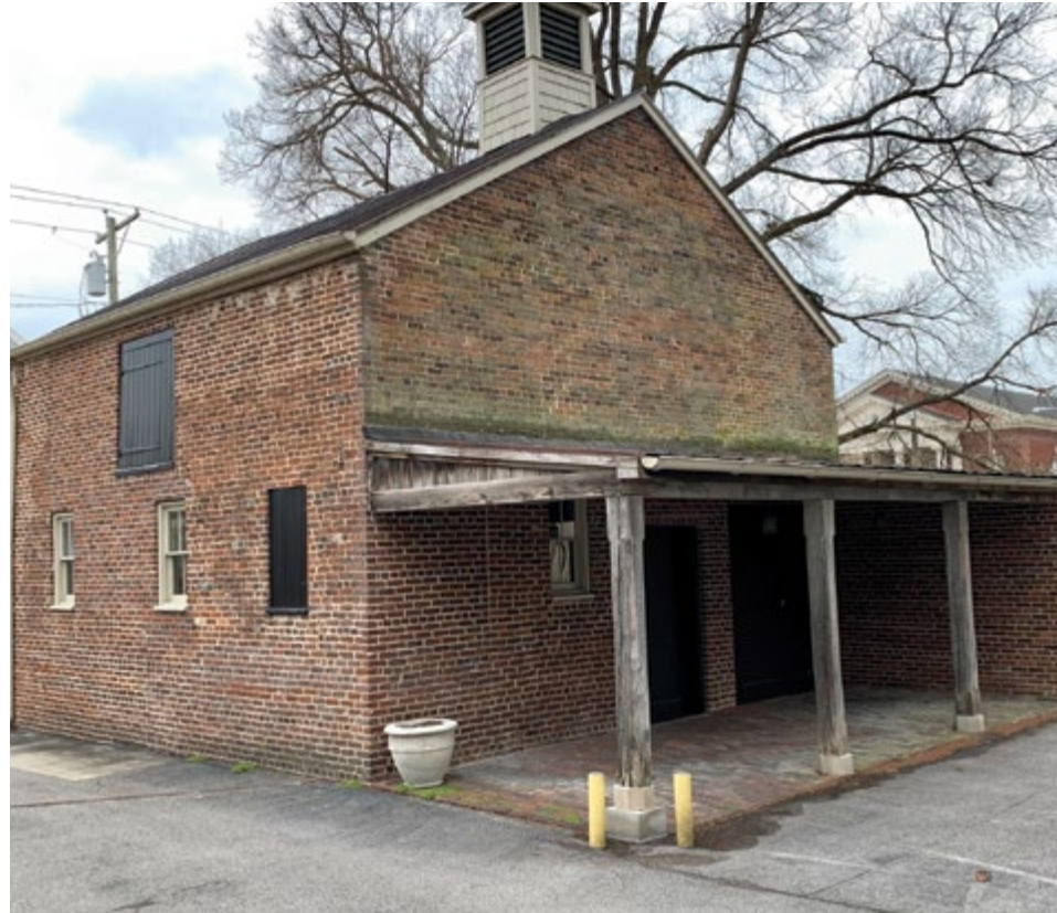
Constructed around 1830-40, the carriage house was built to house the family carriage and carriage horses. The building contains two carriage doors, one on Second Street and one on the back side of the carriage house. This allowed the carriage to pull forward into the house and out of the house without attempting to back up the horses. Note the second-floor door where hay, grain, and straw was unloaded into the loft.
