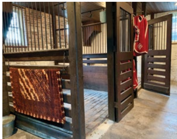
The carriage house has two stalls, where the horses were kept while unhitched from the carriage. Each stall has a hay drop where hay was fed to the horses from the storage room above.
