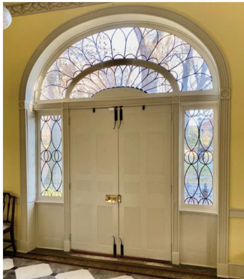
The front door of Hopemont, distinguished by its fanlight and pocket shutters, welcomed guests into this Federal home built in 1814.
