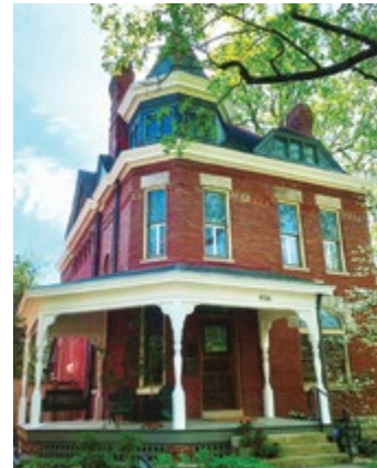
State tax credits of $15,000 for exterior repairs to this c1889 home in Lexington's Fayette Park included masonry and limestone foundation repointing and repair and rebuilding of two chimneys.
