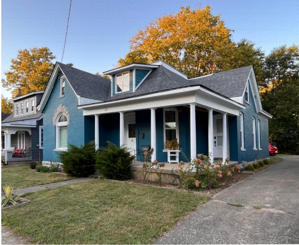
Image 1: South and east elevations
