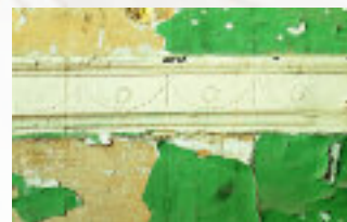
Original molding detail
